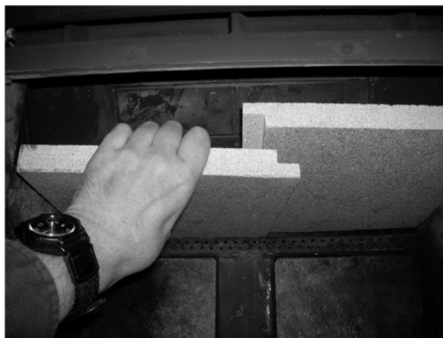
Figure 16 - Removing/Replacing the Baffle for Inspection
